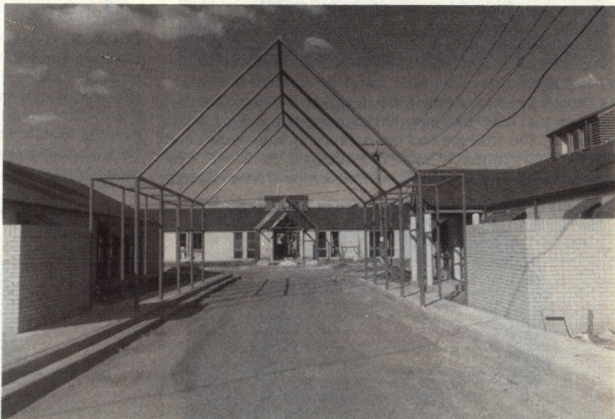
New HQ MP Centre at Green Hills
